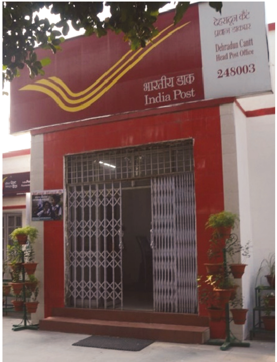
Post Office, Garhi Cantt
