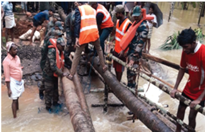
A makeshift bridge being constructed at Cannanore District
